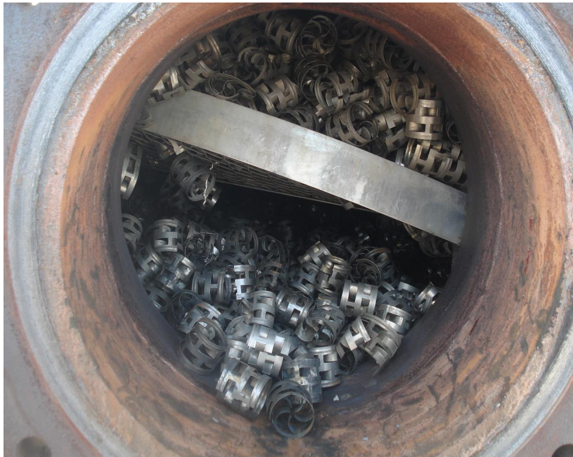
Figure 5: Displaced packing support grid after high liquid level in reboiler
