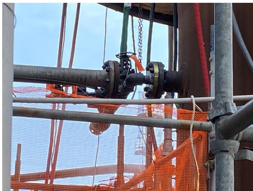
Figure 2: A close coupled wash connection (no valve on vessel nozzle)
